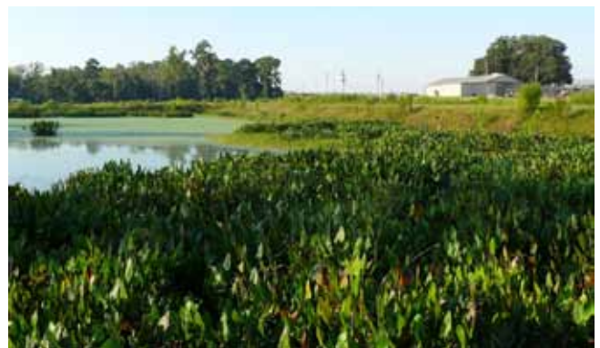
Figure 4. Constructed wetlands can remove nutrients, pathogens and heavy metals from runoff. Photo provided by Sarah A. White.
