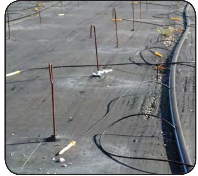
Figure 35. If not kept out of pathways, emitters can become a tripping hazard for workers
