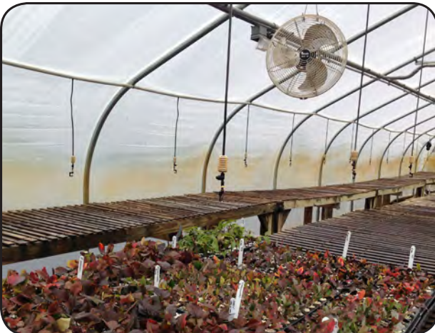
Figure 15. Iron in water can leave a residue on plants as well as the greenhouse structure
