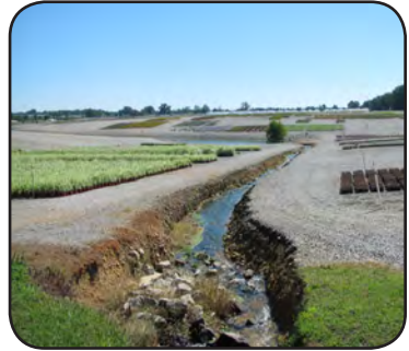
Figure 52. Use the natural slope of the land to passively guide water to a containment structure
