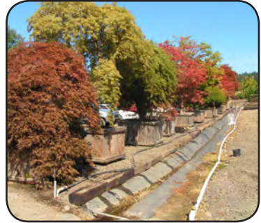
Figure 54. Conveyance ditches carry water to containment structures
