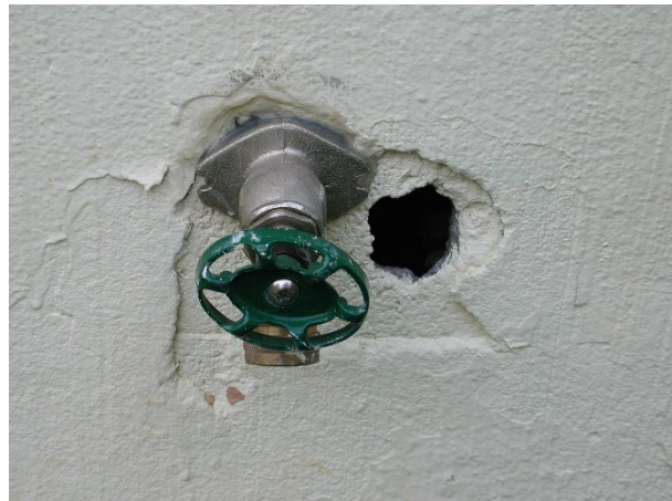
Figure 3. Holes in the foundation and around plumbing, conduit and wires should be sealed to prevent pest entry.
