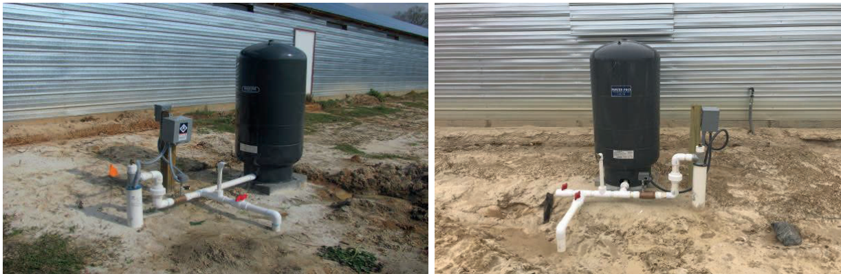
Figures 1 and 2. Can rainwater off the poultry house roof find its way down the wellhead and into the aquifer below?
