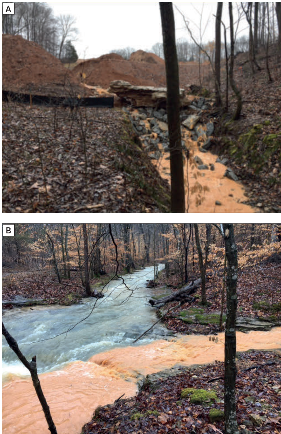
Figure 3. An example of (A) sediment laden stormwater runoff from a construction site and (B) the resulting downstream sediment plume at a stream confluence. Stormwater discharges from construction sites are prohibited from causing visible sediment plumes.
