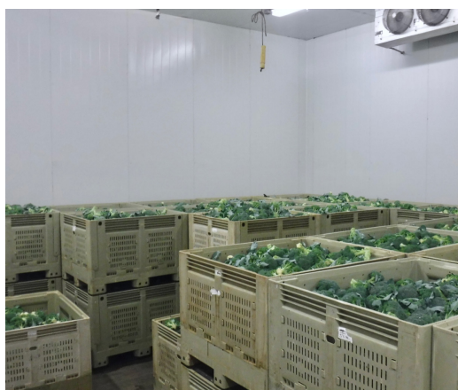
Figure 20. Room cooling of broccoli. Note the mist nozzle above the broccoli. Some growers add mist nozzles to their cold room to minimize dehydration.
