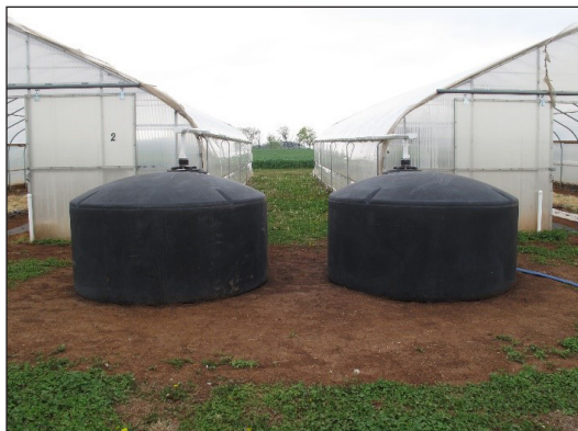
Figure 2: Collection tanks that were used to store rainwater. The holding capacity of these tanks was 1,100 gallons each. The dark color was chosen to inhibit microbe growth within the tank.
