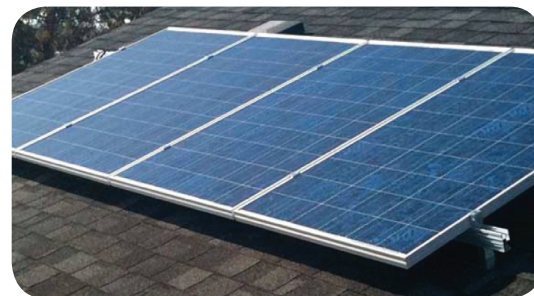
Multi-crystalline silicon PV panels on a rooftop. Four, 250-watt PV panels = 1,000 watts = 1 kilowatt (kW). Together, they produce 1 kWh of electricity per hour in direct (peak) sun. If the panels get four hours of direct sun, the system may produce 4 kWh that day.
